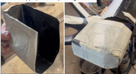
1st BB end cap part, adhesive tape for edge trim lines
